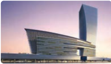
U Bora Tower – Business Bay, Dubai, UAE Air Handling Units (AHUs) Condensing Units
