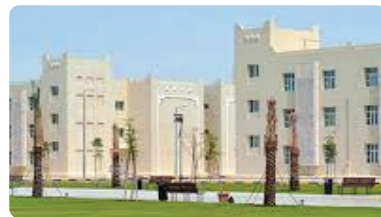
Labour City, Doha, Qatar 50 Kw Tank Chillers – 216 Qty
