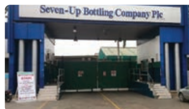
Seven-Up Bottling Company Plc, Nigeria Condensing Unit Air Handling Units (AHUs)
