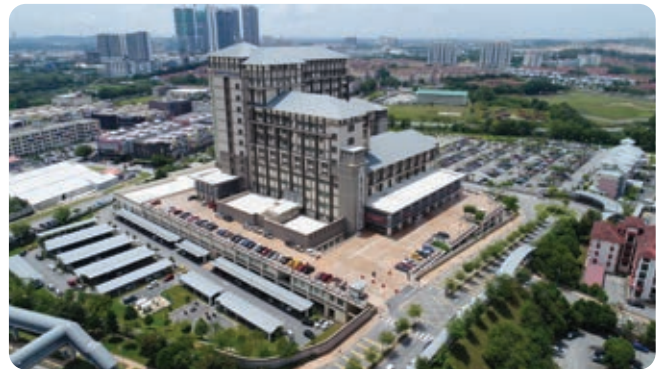
SHAH ALAM HOSPITAL, MALAYSIA
