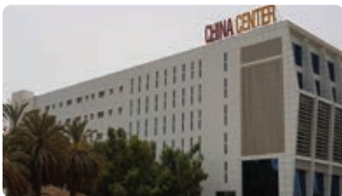
China Center, Seeb, Sultanate of Oman All Inverter VRF System – 1340 HP
