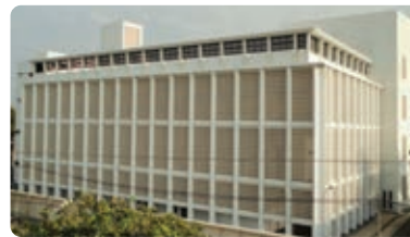
Jaffna Hospital, Sri Lanka Air Handling Units (AHUs) Condensing Units
