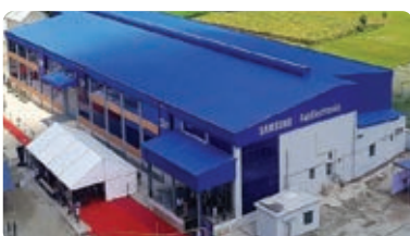
Fair Distribution, Dhaka, Bangladesh DX Chiller Air Handling Units (AHUs)
