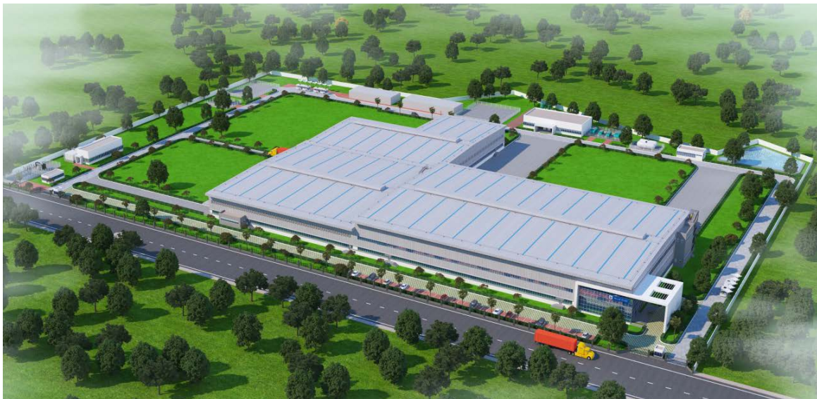
Bird's-eye view of Phase 1 of Blue Star Climatech Limited's Sri City Plant
