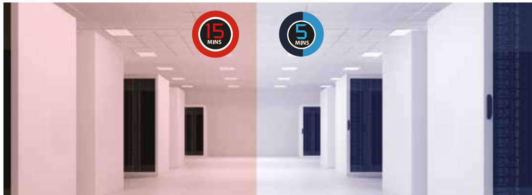
Conventional Screw Chillers
