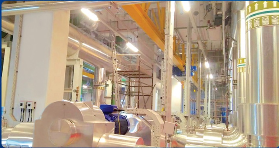
Al Bayt Stadium, Energy Centre Project, Qatar
