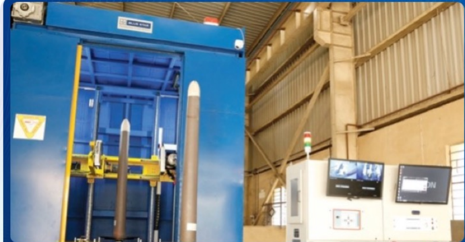
Tata Refractory Limited, Odisha
